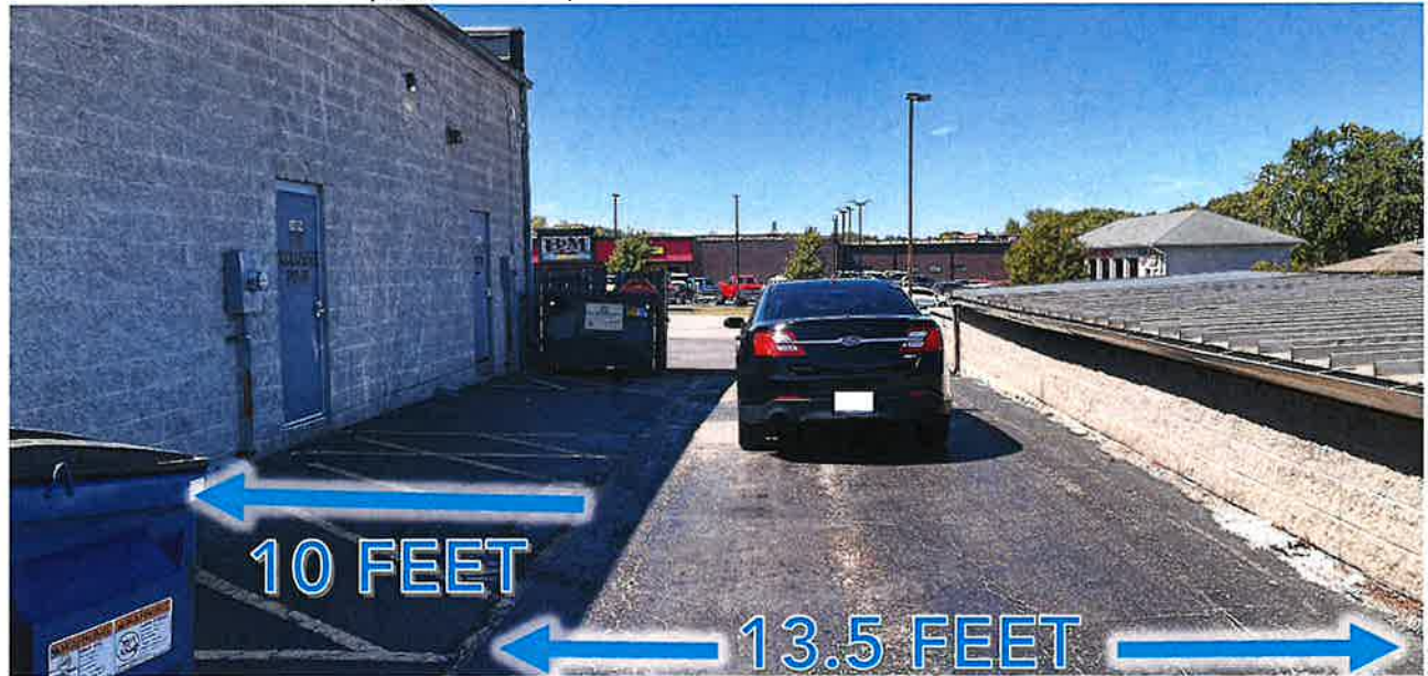
Vehicle traffic in the rear of this shopping center
