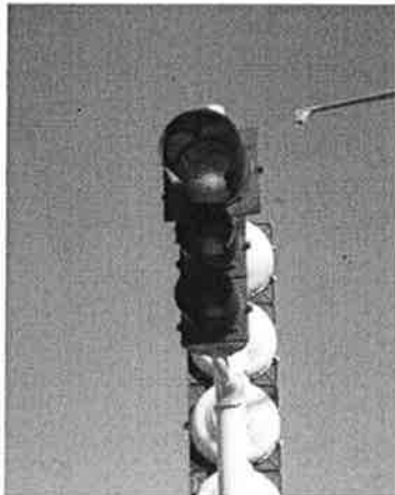
12 inch red and 8 inch yellow and green ball at some approaches of 167 th St & Cicero Ave.
